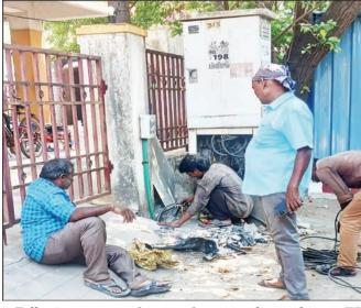
Following outage of power for more than 6 hours, EB workers were seen replacing a portion of the damaged power cable connecting two pillar boxes on Kothandaramar Temple Street (West Mambalam). The photo was taken at 2 p.m on March 13.
