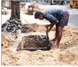
Following complaints of water contamination, Metrowater workers dug a pit to locate the leakage in the Metrowater pipeline in Giri Road (West Mambalam) on March 6.
