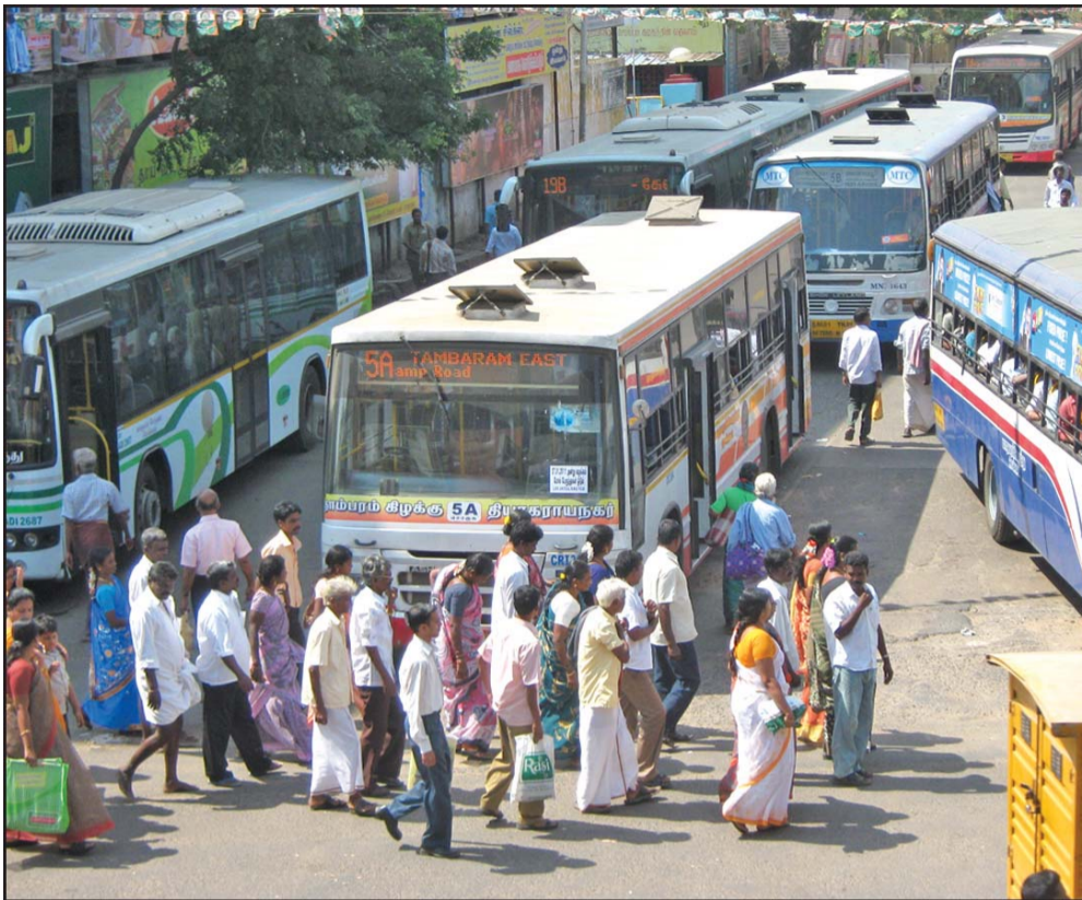
The feasibility report envisages a two-level bus station. The ground level will be remodelled to efficiently regulate bus movement. There will also be public utilities such as ATMs and toilets. The facilities will be built through the Build Operate Transfer (BOT) model.
